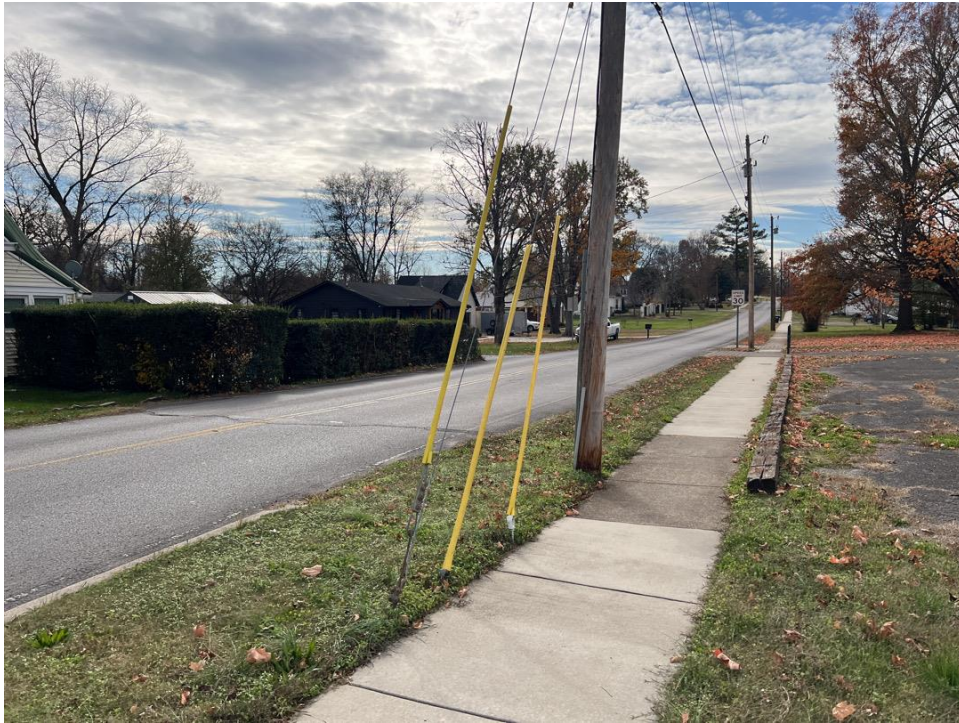
Unsignalized Intersection Deficient pavement markings, minimal shoulder.
