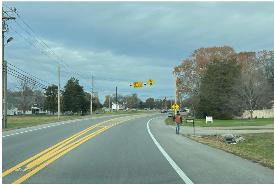
Pedestrian walking along the shoulder Missing pedestrian facilities along the segment.
