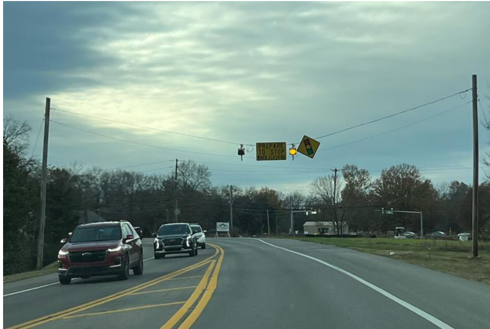
Advanced traffic signal warning infrastructure Upgrade to modern equipment.
